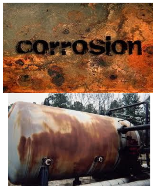
Figure 3. Corrosion of equipment surfaces.
