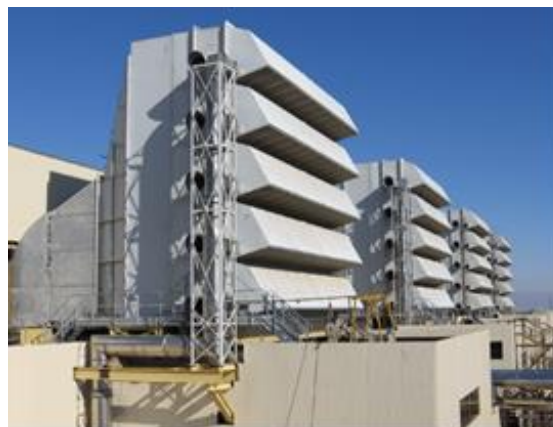
Figure 2. Air Intake system
